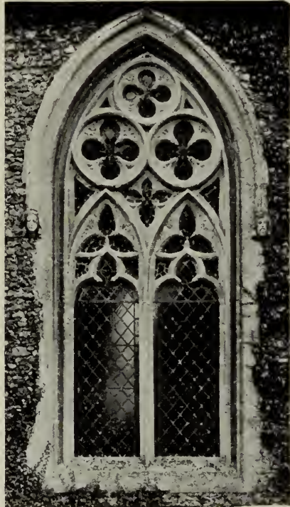
134. A SOUTH-AISLE WINDOW, RICKINGHALL INFERIOR, SUFFOLK
